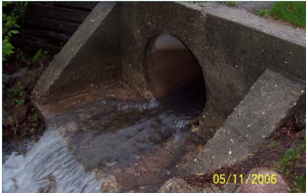
Stormwater System Entry Point into Boardman River
