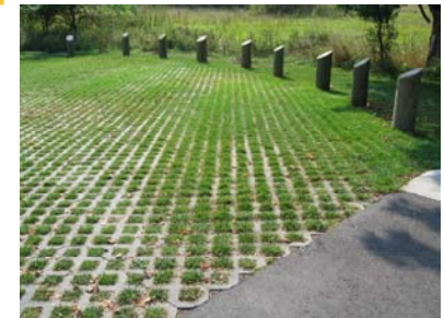
Grand Traverse Commons - Utilize porous/pervious pavement, where appropriate. (Below) - Impervious area on Elmwood Ave.
